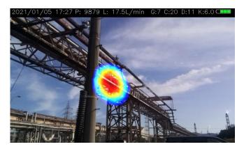
The compressed air leak from the pipe in high place out of reach is found.
