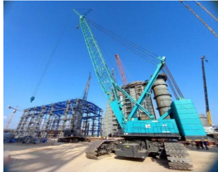
Crawler Crane 250 T
