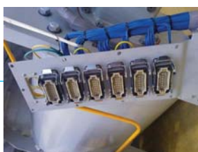
■ High-tension switch cabinet
