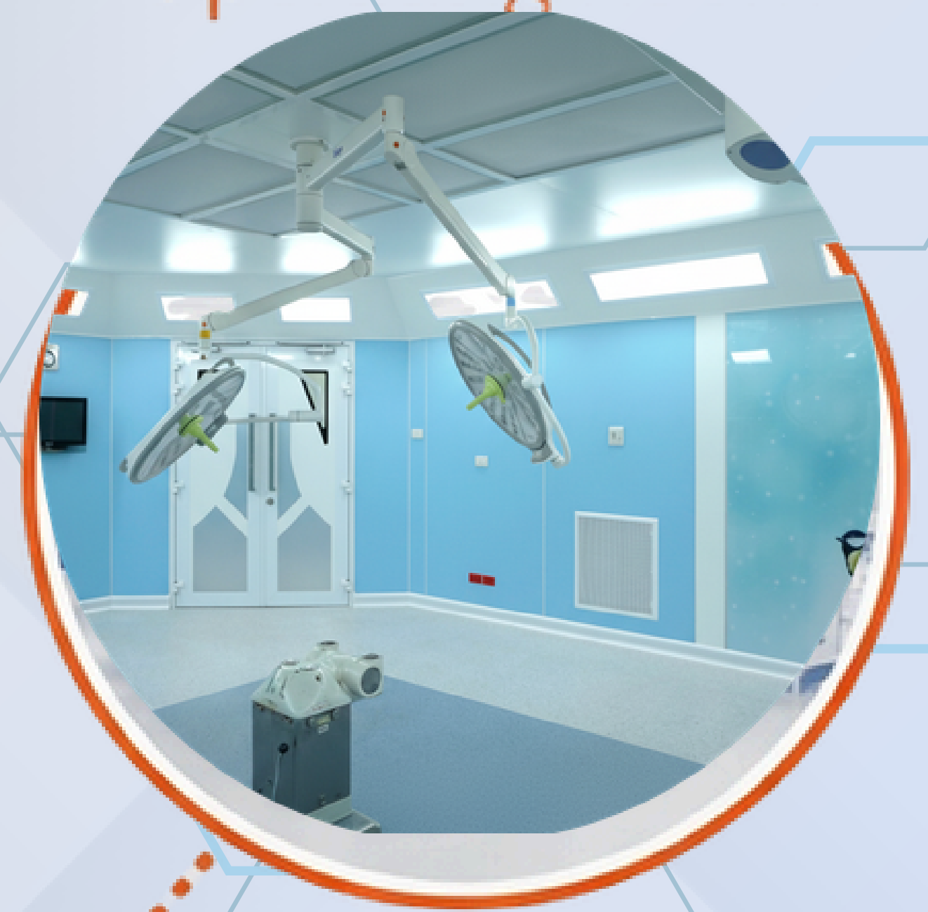
Hospital Operating Room
