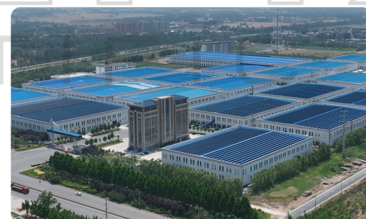
BIOBASE Juancheng County Medical Equipment Industrial Park
