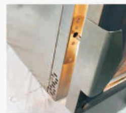
Electromagnetic door lock
