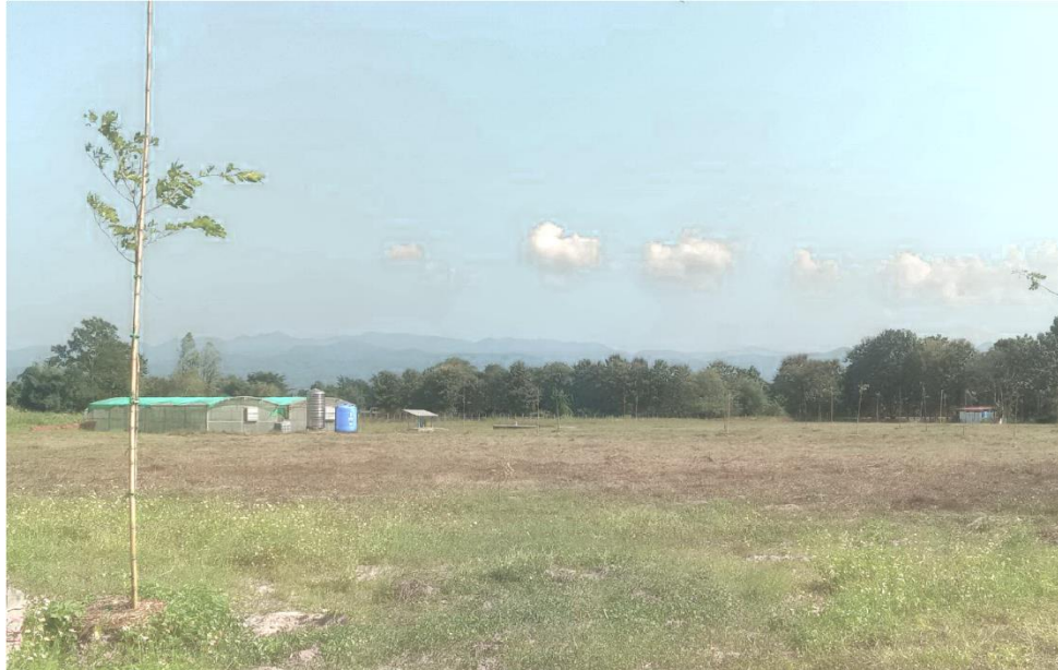
Eastern View of Golden Immortal Hotspring Project.
