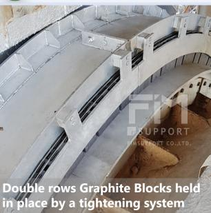
► **Self adjustment** seal is always fitted with rotating part of kiln shell, nearly zero gap in between is maintained.
