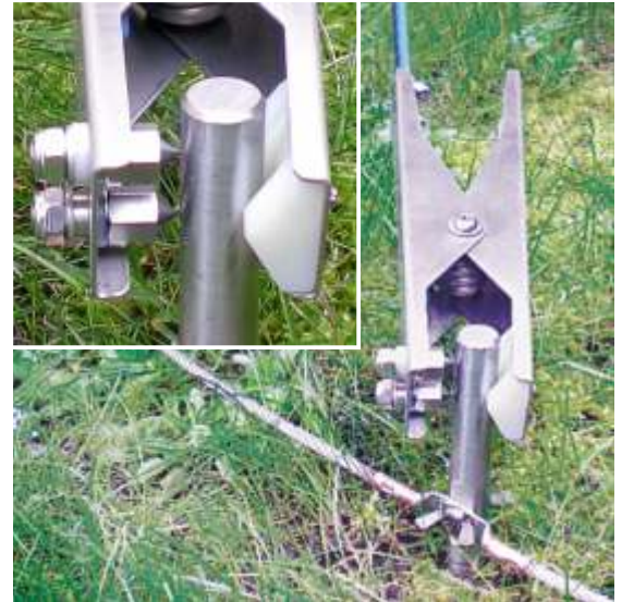
Quick release static grounding clamp supplied with the Earth-Rite II MGV attached to buried rod.
