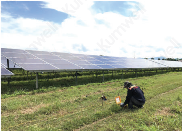
THAILAND : Super Energy Solar Farm
