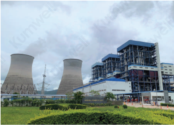
THAILAND : HPC Power Plant
