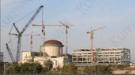
CHINA : 6100 MW YANGJIAN NUCLEAR POWER PLANT
