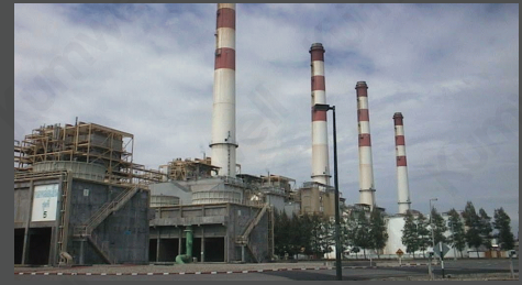
THAILAND : PTT GASSEPARATION PLANT
