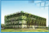
The Netherlands Bytesnet, Colocation 6 MW
