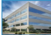
India Leading Colo Data Center 28 MW Telecom Data Center 7 MW
