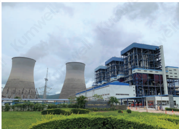
THAILAND : HPC Power Plant
