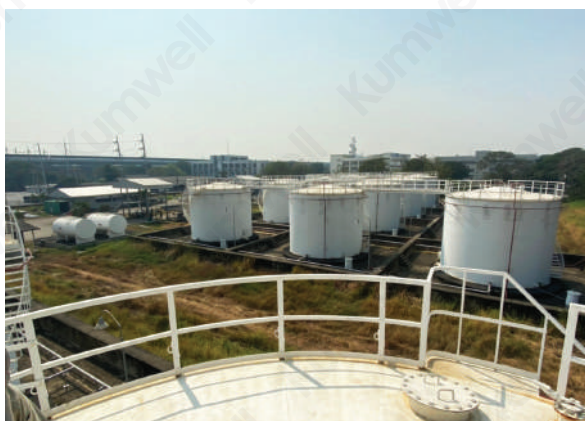
THAILAND : Air Force Fuel Depot
