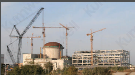
CHINA : 6100 MW YANGJIAN NUCLEAR POWER PLANT
