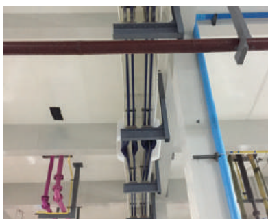
Aluminum busbar installation
