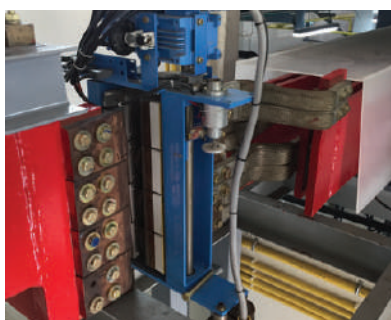
DC Switch installation
