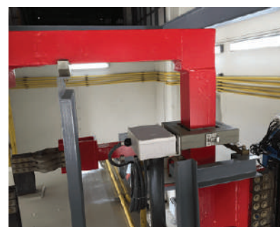
DC Current transducer DynAmp installation
