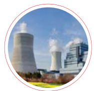
Thermal Power Generation
