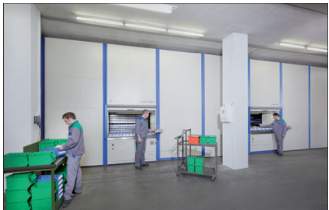
Two Hänel Multi-Space® units each 9.57 m wide constitute the central store for the production hall
