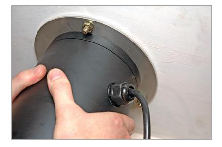
Cut the multicore cable to the desired length and re-test the connections.
