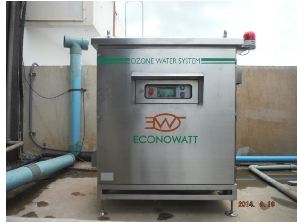
• Pitsanuvej Hospital (Pitsanulok)
