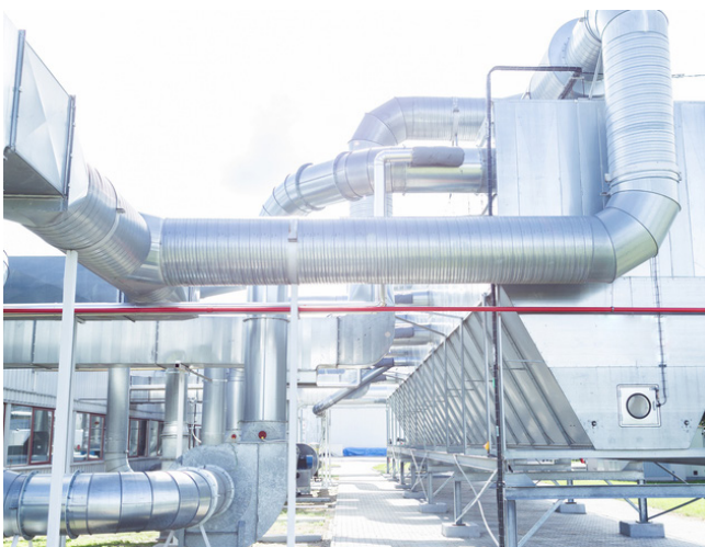
Dust collector in a woodworking factory
