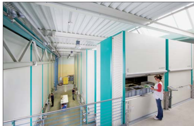
Depending on the height of the Hänel Lean-Lifts®, access points can be installed on different floors. Several people can use the Hänel Lean-Lift® simultaneously at different positions and levels
