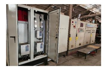
➤ Project to reduce the time for grinding raw materials in the ceramic clay preparation process. The goal is to reduce electrical energy in the raw material grinding process by more than 10%, resulting in savings in both energy and an increase in production capacity without adding additional machinery.
