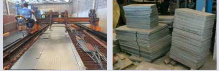
CNC machine steel cutting parts
