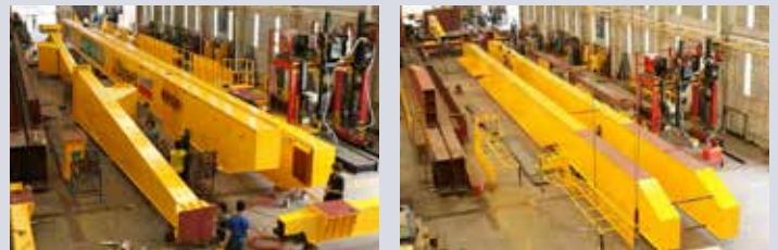
Pre structure assembly
