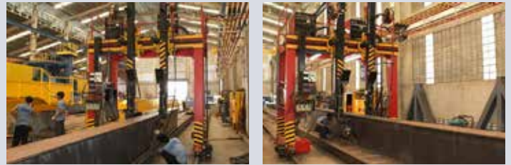
Box girder weld machining
