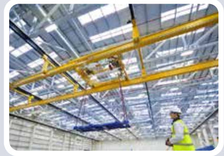
Underhung Cranes : Double Girder
