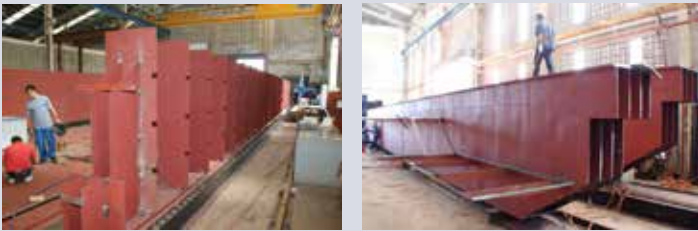
Fabrication box girder profiles
