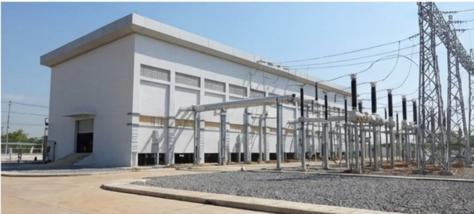
230kV GIS Substation - EGAT Ayuthaya
