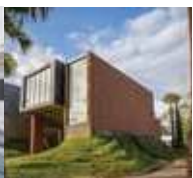
THE VICTORY BY ANDAMAN ASSET SOLUTION
