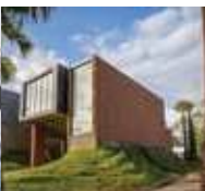
THE VICTORY BY ANDAMAN ASSET SOLUTION
