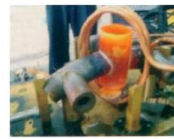
水龍頭焊接 Welding sanitary ware. tap
