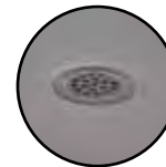
Slope with 2-inch sink-type drain.
