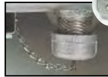
A stainless chain secures the threaded cap for 1-1/2" pipe drain.
