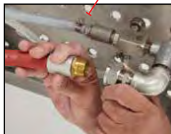
Connects to garden hose with quick-disconnect.
