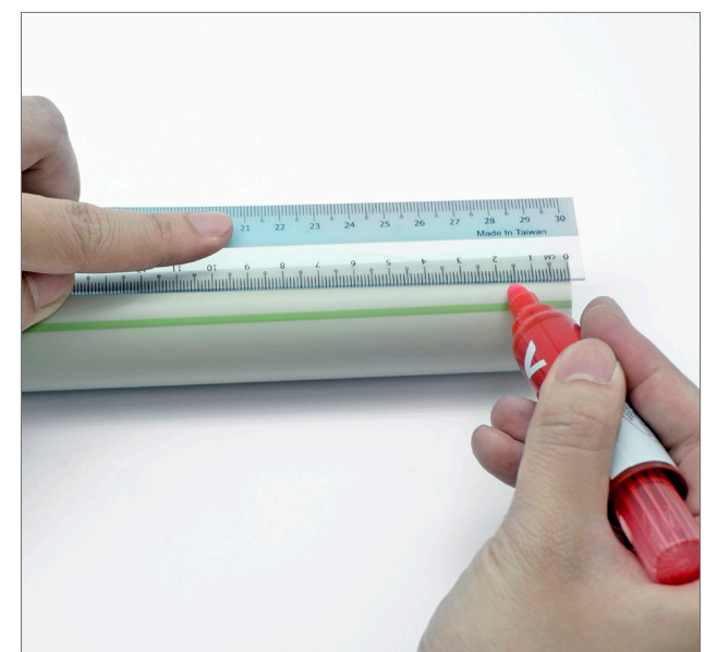
Mark the pipes
