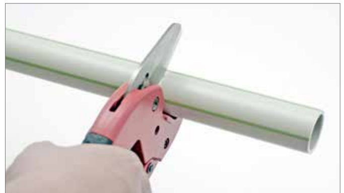
Fig. 8-4 Cut the pipes
