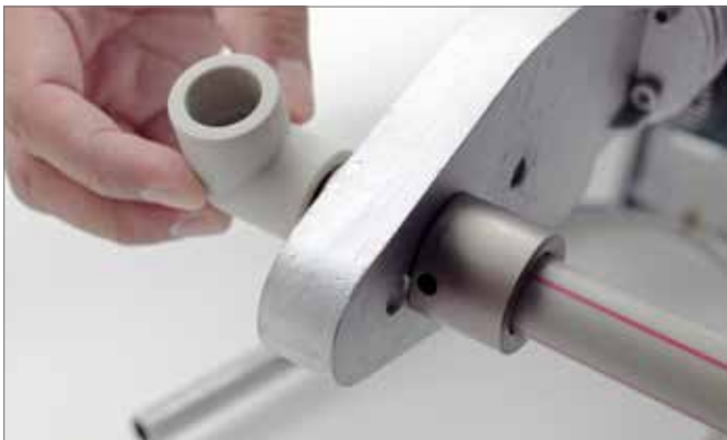
Fig. 8-6 Heat the pipe and fittings
