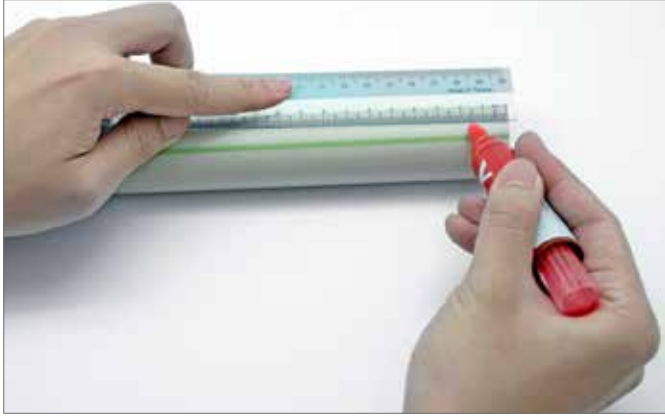
Fig. 8-5 Mark the pipes
