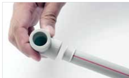
2 Fuse the fitting
