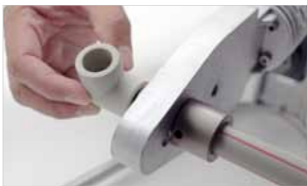
1 Heat the pipe and fitting
