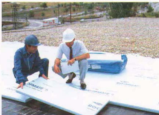
Ballasted Upside-Down roofing
