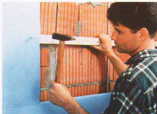
Fixing of insulation boards
