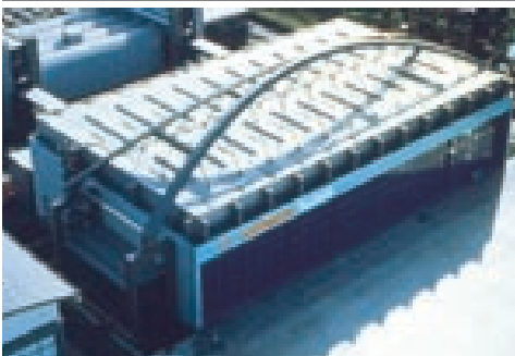
▲ Jumbo aircraft hangar, Hamburg Airport
