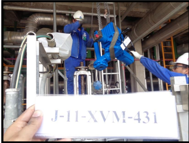
Installation Actuator at Site
