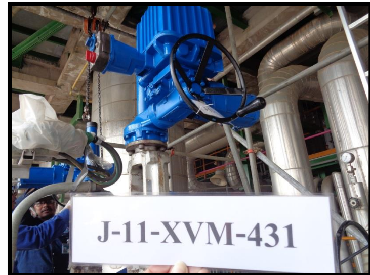
Installation Actuator at Site
