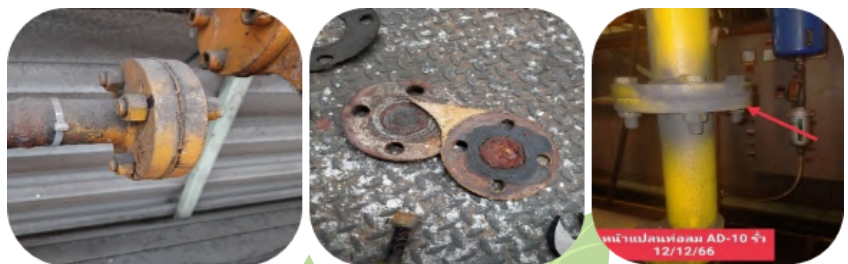
Change the gasket air pipe
