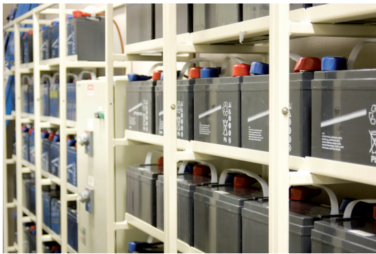
60-120kVA adjustable number of battery : 28/29/30/31/32pcs
