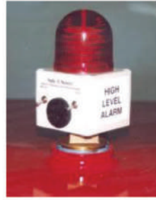
Tank High level alarm
