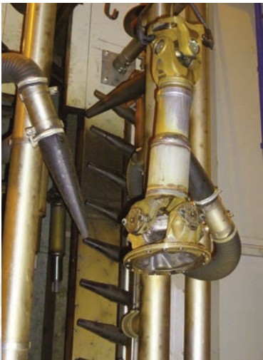
Drying automotive drive shafts
