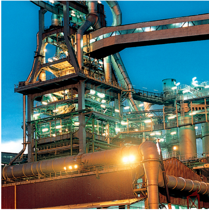
Industrial application: Refinery
