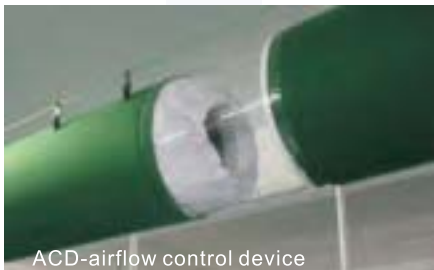
ACD-airflow control device
