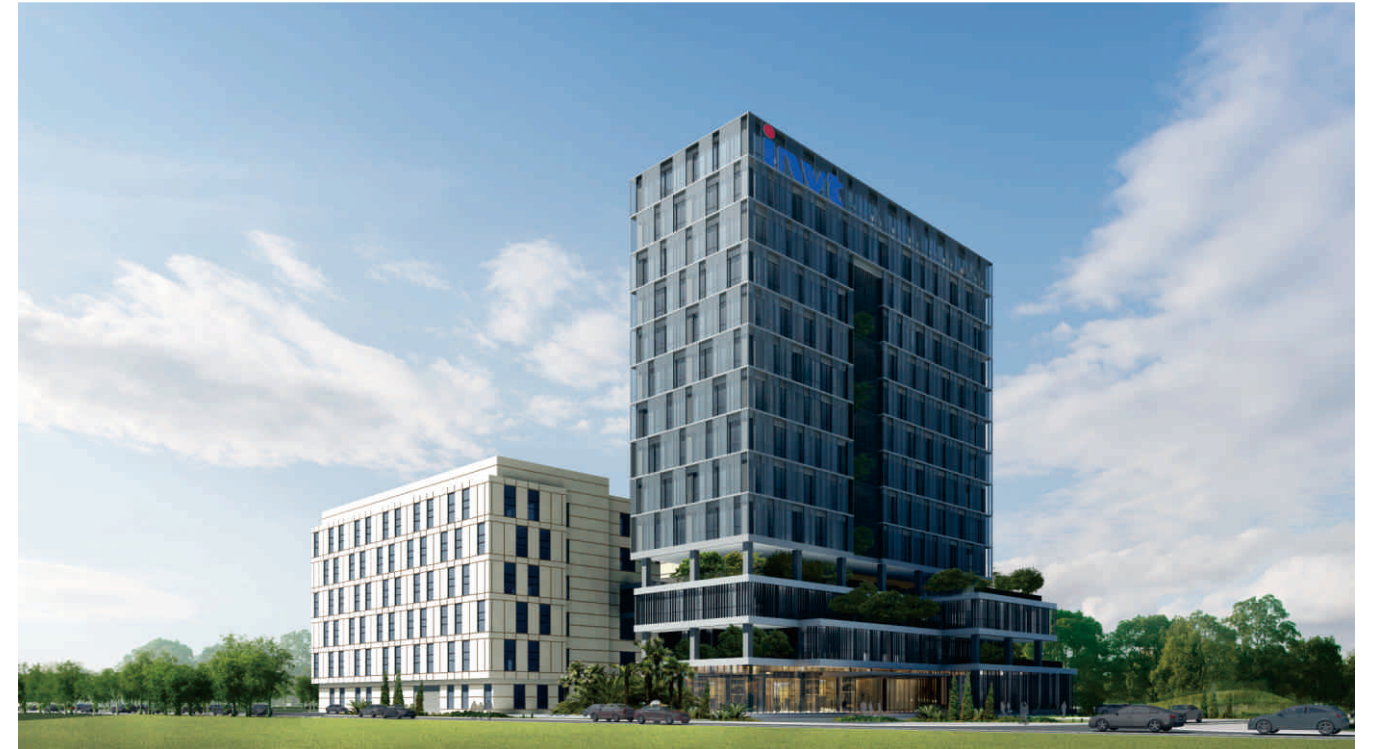
Shenzhen Industrial park
