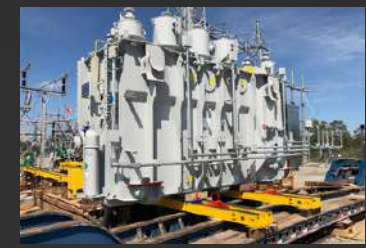
Transformer / Jacking and Skidding
