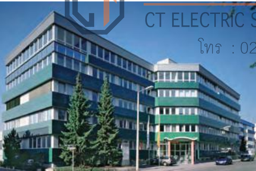
Lapp-Center in Stuttgart
