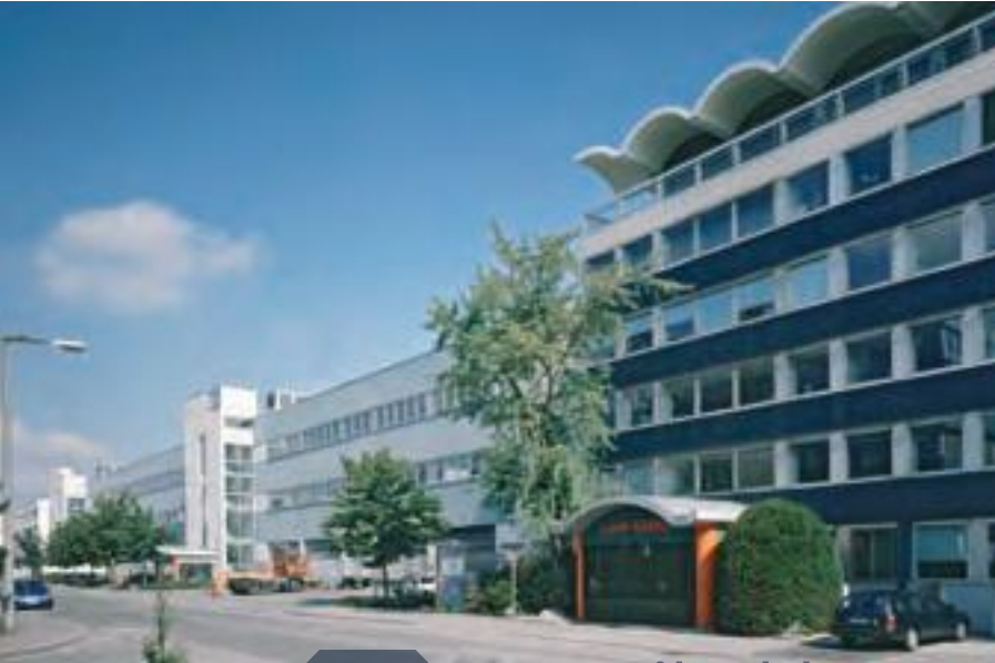
Headquarters in Stuttgart
