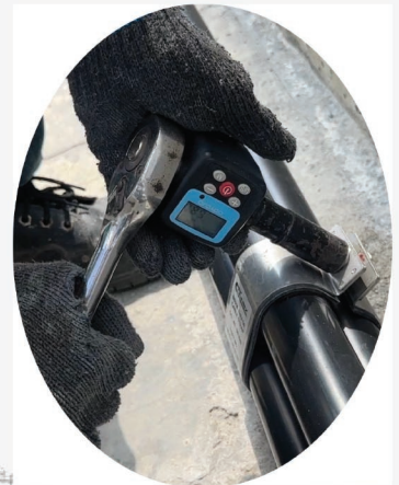
6. TIGHTEN MOUTH BOLT NUT
