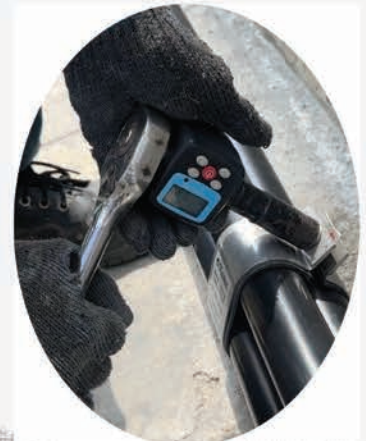
6. TIGHTEN MOUTH BOLT NUT
