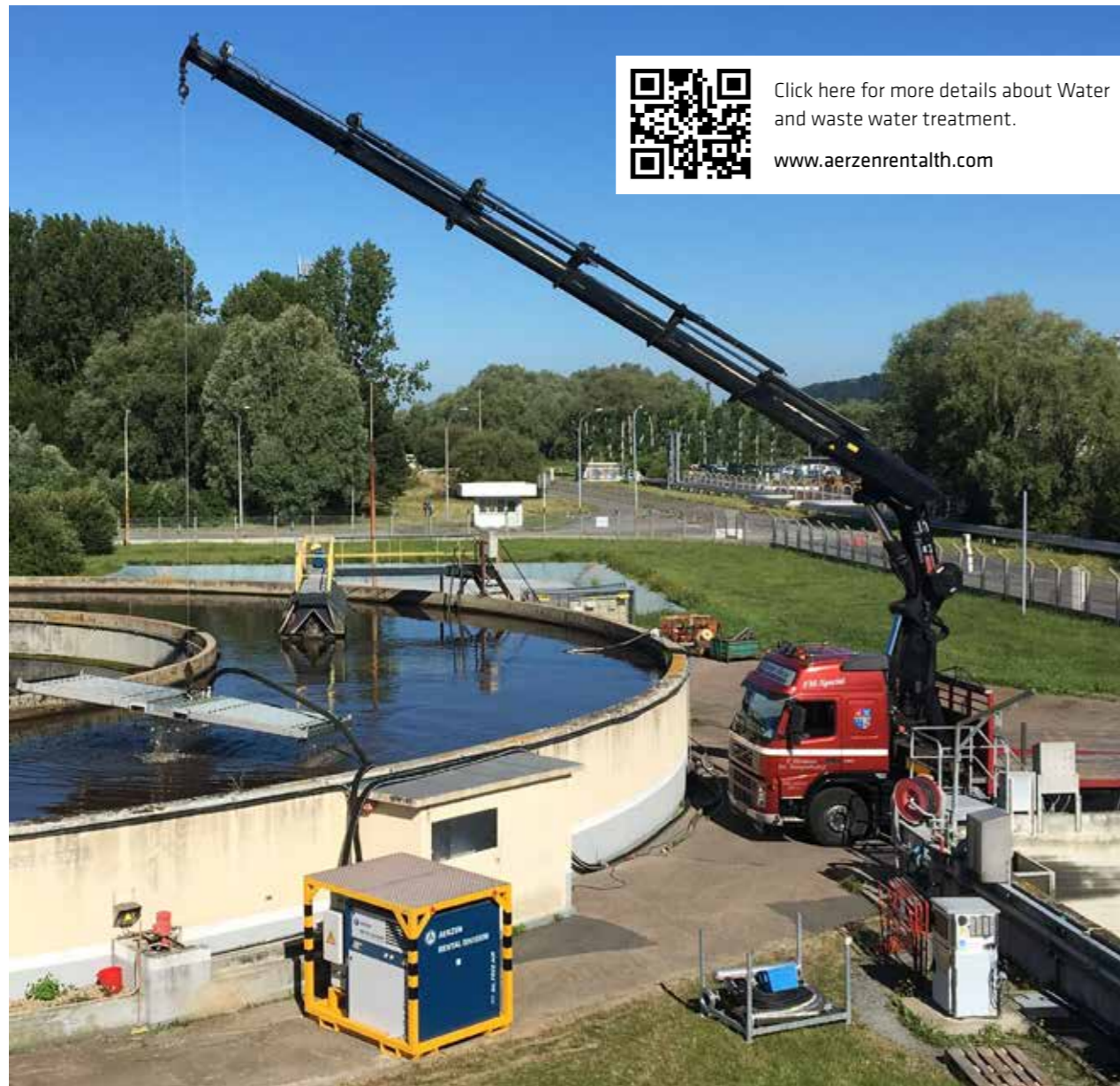
Micro biology was threatened to die. Aerzen rental delivered a complete temporary aeration unit installed within 48 hours.
