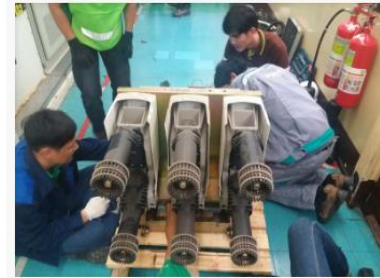
Mitr Phol Replace Truck Evolis Breaker
