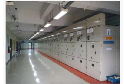
Motor & Switchgear & Installation
