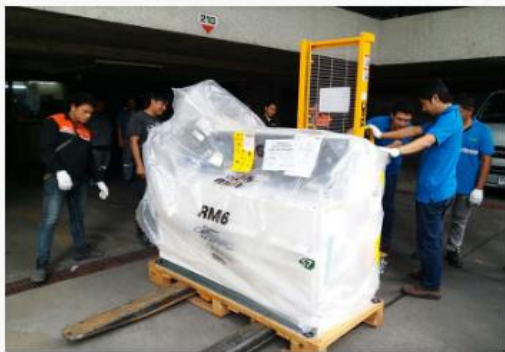
RMU Installation Sasin
