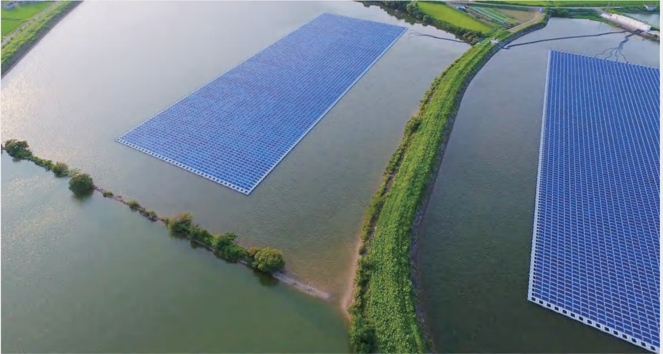
THAILAND 8MW FLOATING PHOTOVOLTAIC POWER PROJECT
