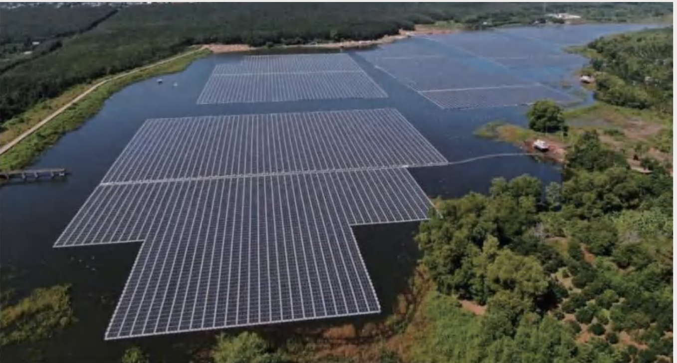
CHINA 30MW FLOATING PROJECT REFERENCE
