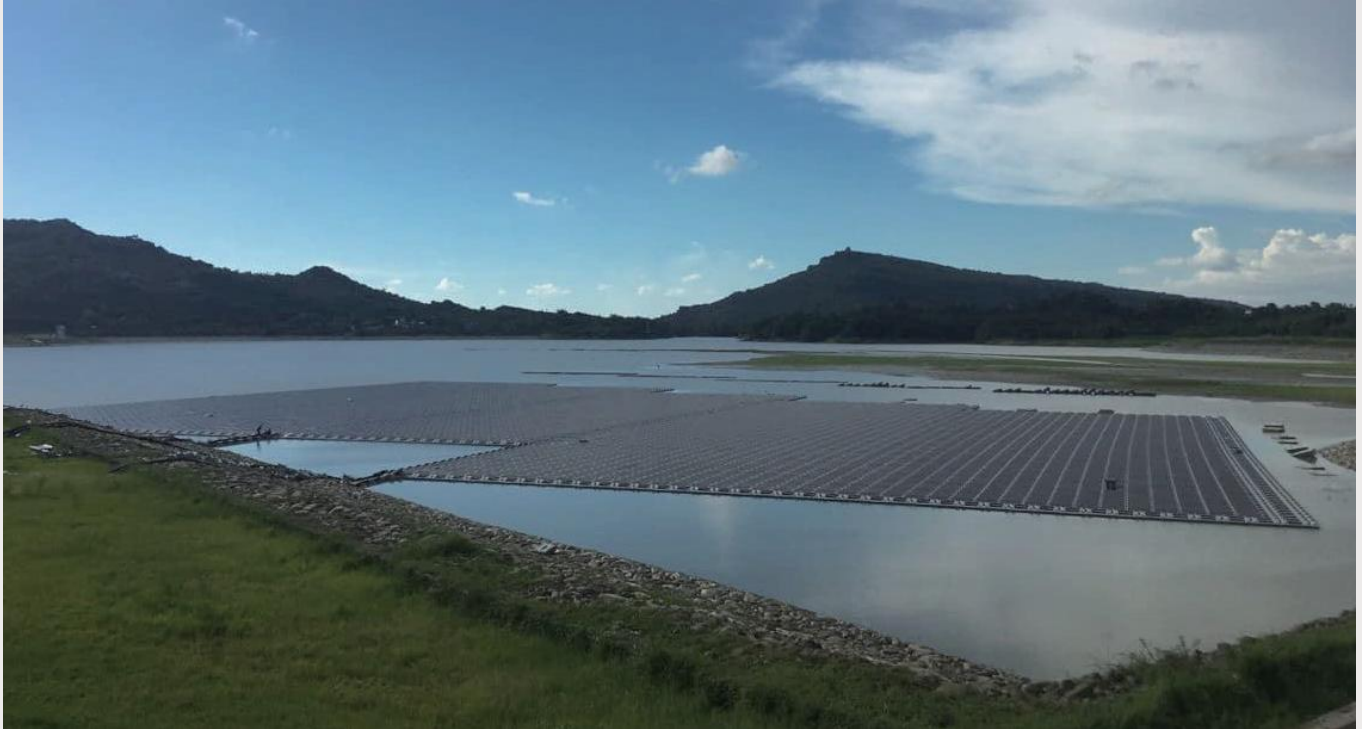
CHINA 300KW FLOATING PROJECT REFERENCE
