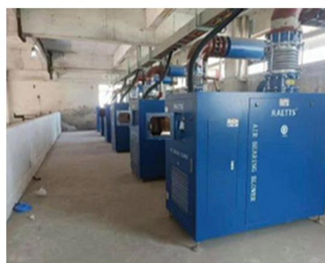
Dyeing, Weaving and Washing Sewage Treatment Project in Zhongshan Huaxing
