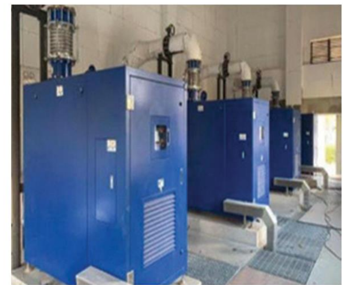
No.1 Sewage factory in Longyang District, Baoshan, Yunnan.
