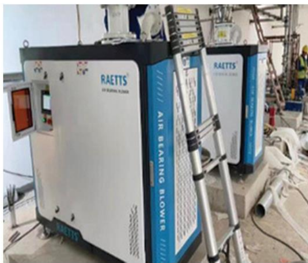
Sewage treatment factory in Guangxi
