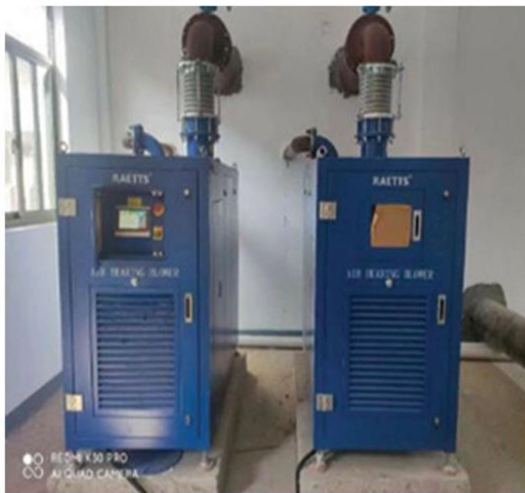
Sewage treatment factory in Changxing Hongqiao
