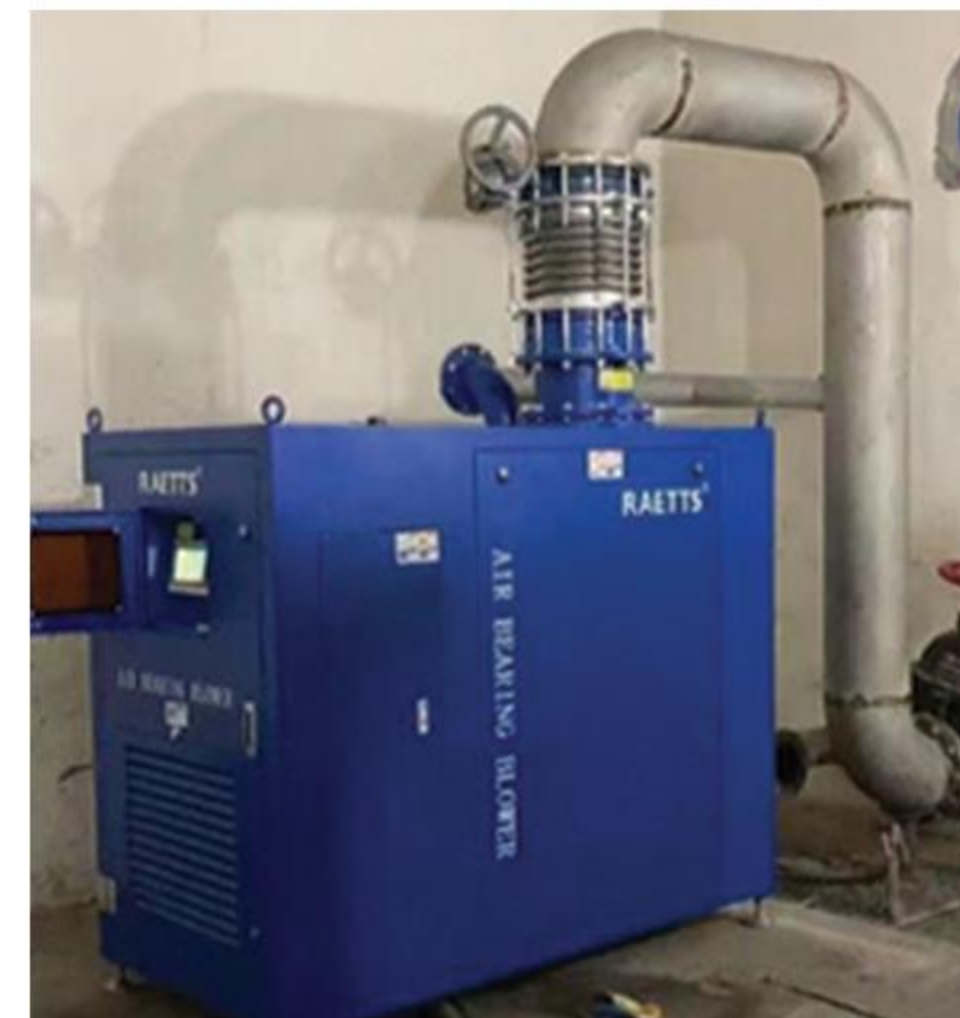
Sewage treatment factory at Guodian Galaxy
