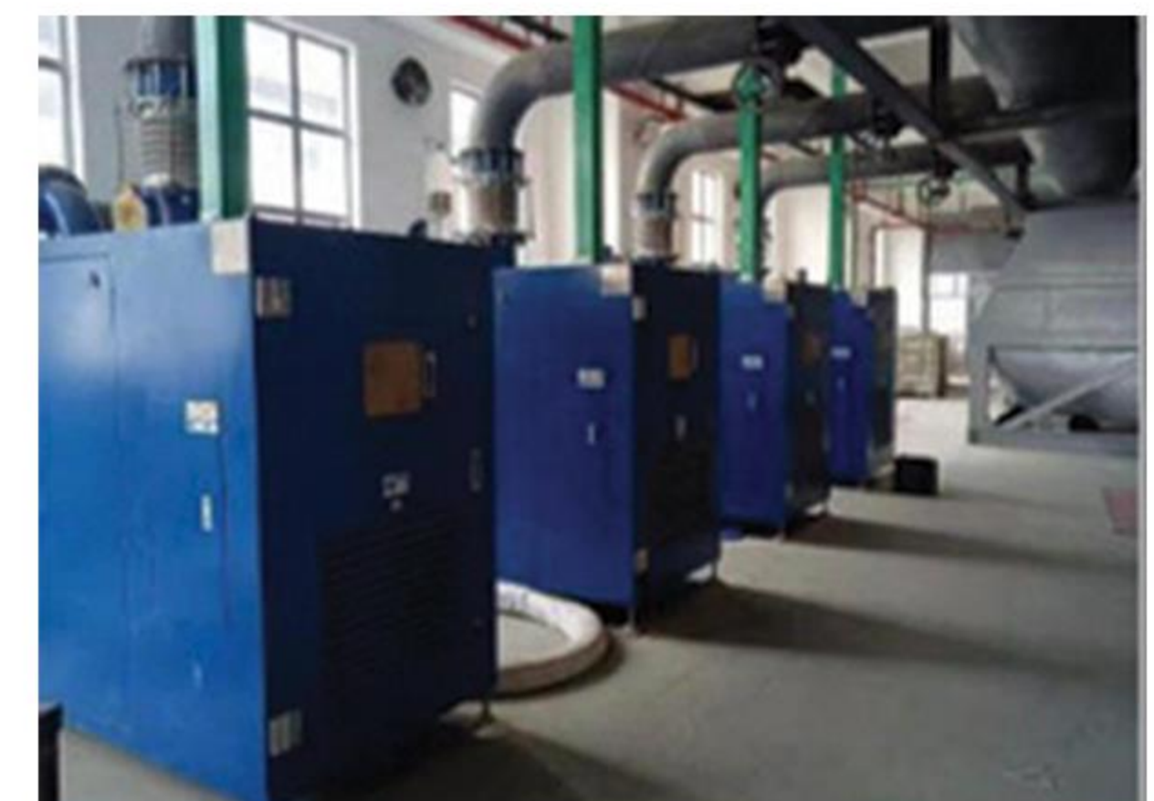
Landfill Leachate Treatment in Mayong, Dongguan
