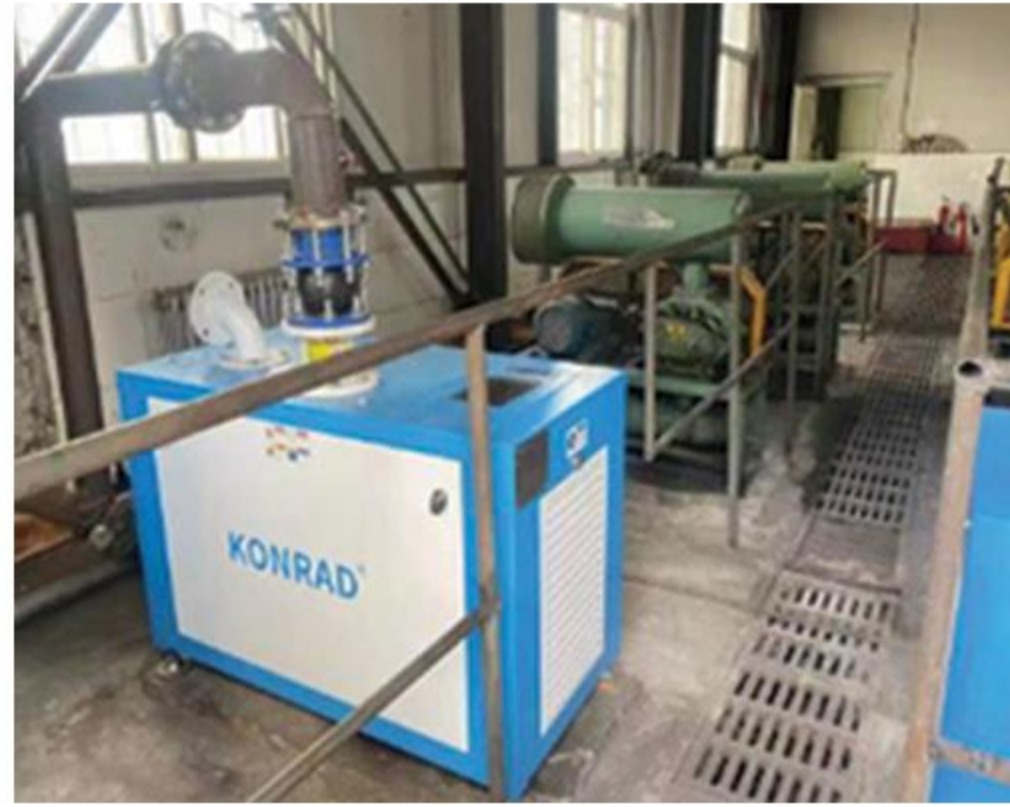
coal industry Sewage treatment factory
