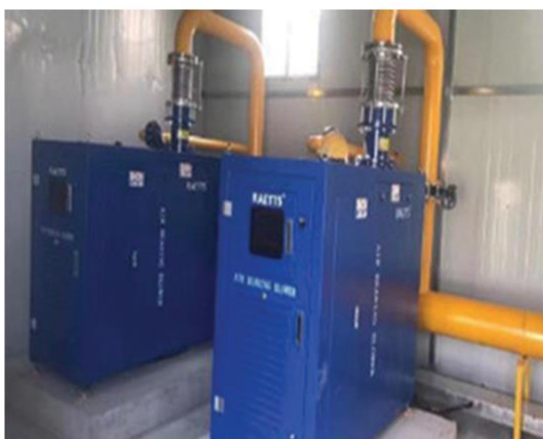
Sewage treatment factory in Huayin City, Shaanxi Province
